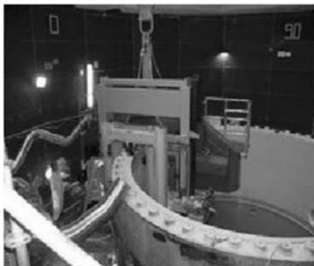
Figure 39: band saw used to cut the reactor vessel in Würgassen
