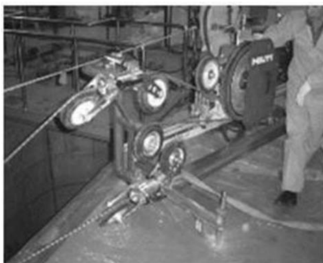
Figure 38: band saw used to cut the reactor vessel in Rancho Seco
