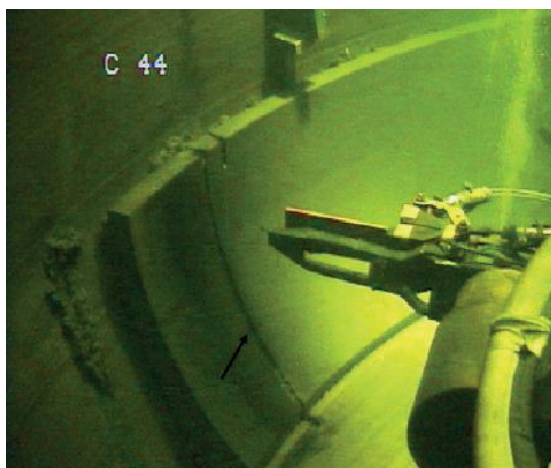
Figure 17: CAMC used to dismantle nuclear facilities
