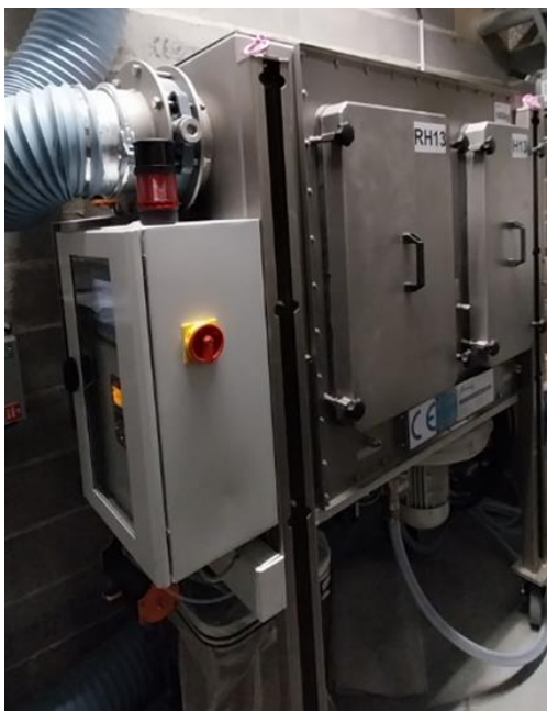
Figure 87: Krantz filtration skid (HEPA filter)
