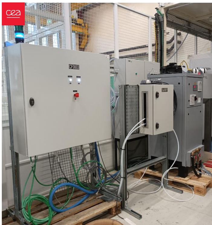
Figure 19: Electrical cabinets et cooling unit
