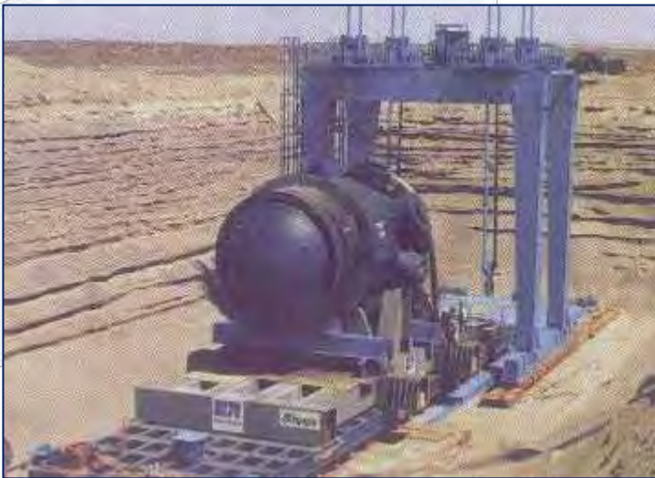
Trojan Reactor final disposal in one piece without segmentation. Source: American Ecology
